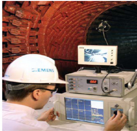
Figure 4: A FAST Gen V generator specialist conducts stator, rotor and wedge inspections conveniently on site, featuring narrated video taping plus high resolution photos
