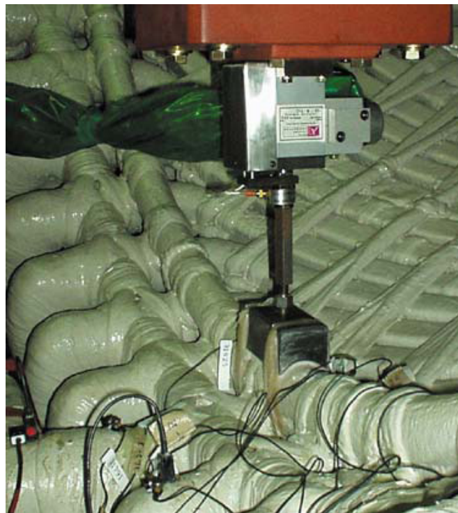
Picture 13: Stator end winding tightening control
