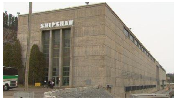
Front gate of the powerhouse
