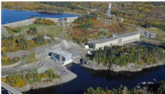
Aerial view of Shipshaw project.
