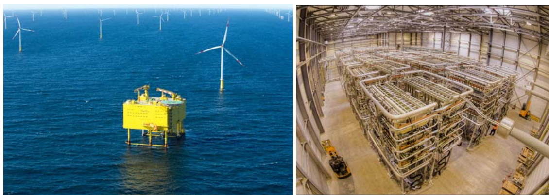
Fig. 1: Offshore VSC platform SylWin1 in operation and converter hall of HelWin1
