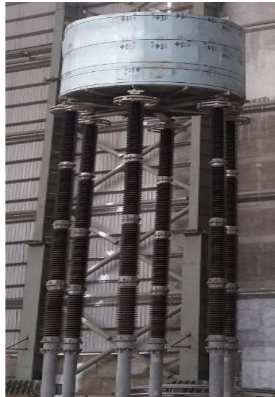
Fig- One coil Smoothing Reactor (75 mH ,2674 A ) at Agra DC hall connected at HV bus (under construction)
