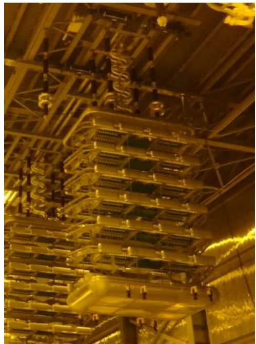
Fig-3, 800 kV Double valve structure of NER-Agra HVDC Project (under construction).
