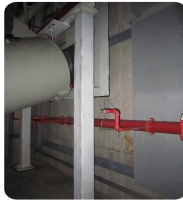
Fig. 14b Bushing with the support frame
