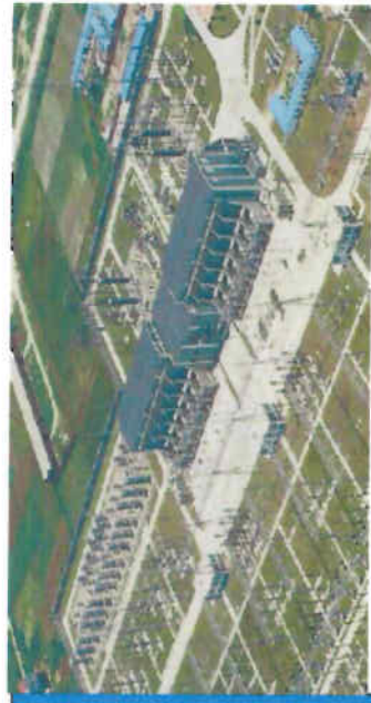
± 500 kV, 3300 MW HVDC
