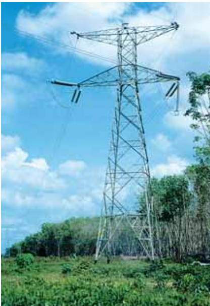
Fig. 5.6.1-1: DC transmission line (bipolar tower 300-kV link)
