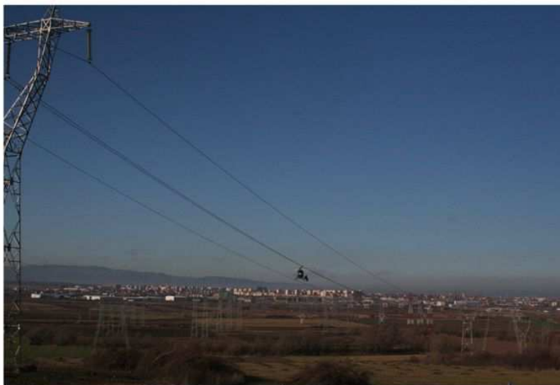
Figure 4. Spacer changing by helicopter with special platform (SC SMART SA line operator)
