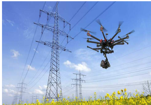
Fig. 2 Advanced monitoring „Heavy” drone
