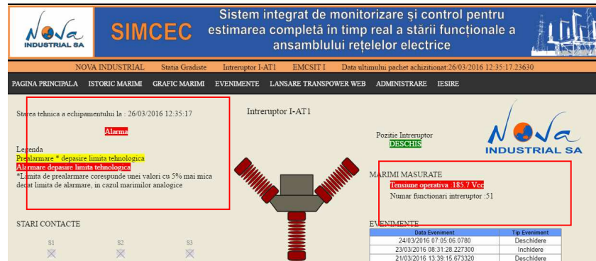
Figure 5. Analysis of the monitored parameters - alarm for the operative voltage for a circuit breaker
